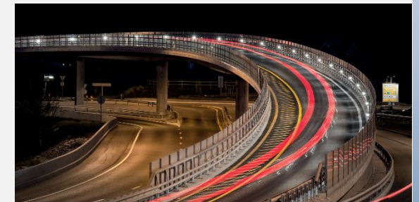
Roads, Transportation & Tunnel
